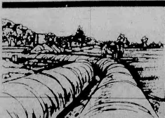
1929 • Wanaque Aqueduct, Pipe laid on ground surface.
